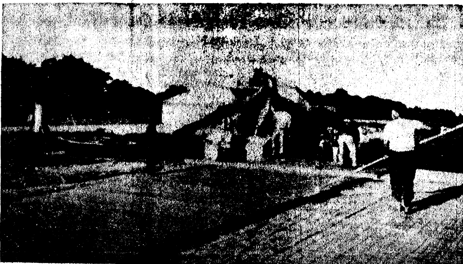
SCHOOL BUILDING ON SCHEDULE: Wednesday, Sept. 1, the concrete slab was poured for the North Sharon Christian School Building. The building 24'x88' is being constructed by National Homes, Inc. The structure is flexible so that additions may be made in stages as they are needed. The building and structure was to arrive Sept. 7 and be erected in one day.
